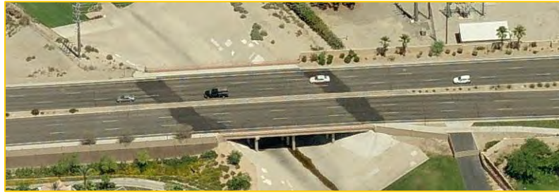
Completed: WSH1 – Washington Street Bridge between Avenues 50 and 52
