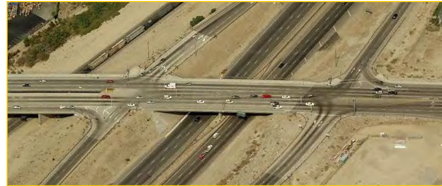
Monterey Interchange at I-10
